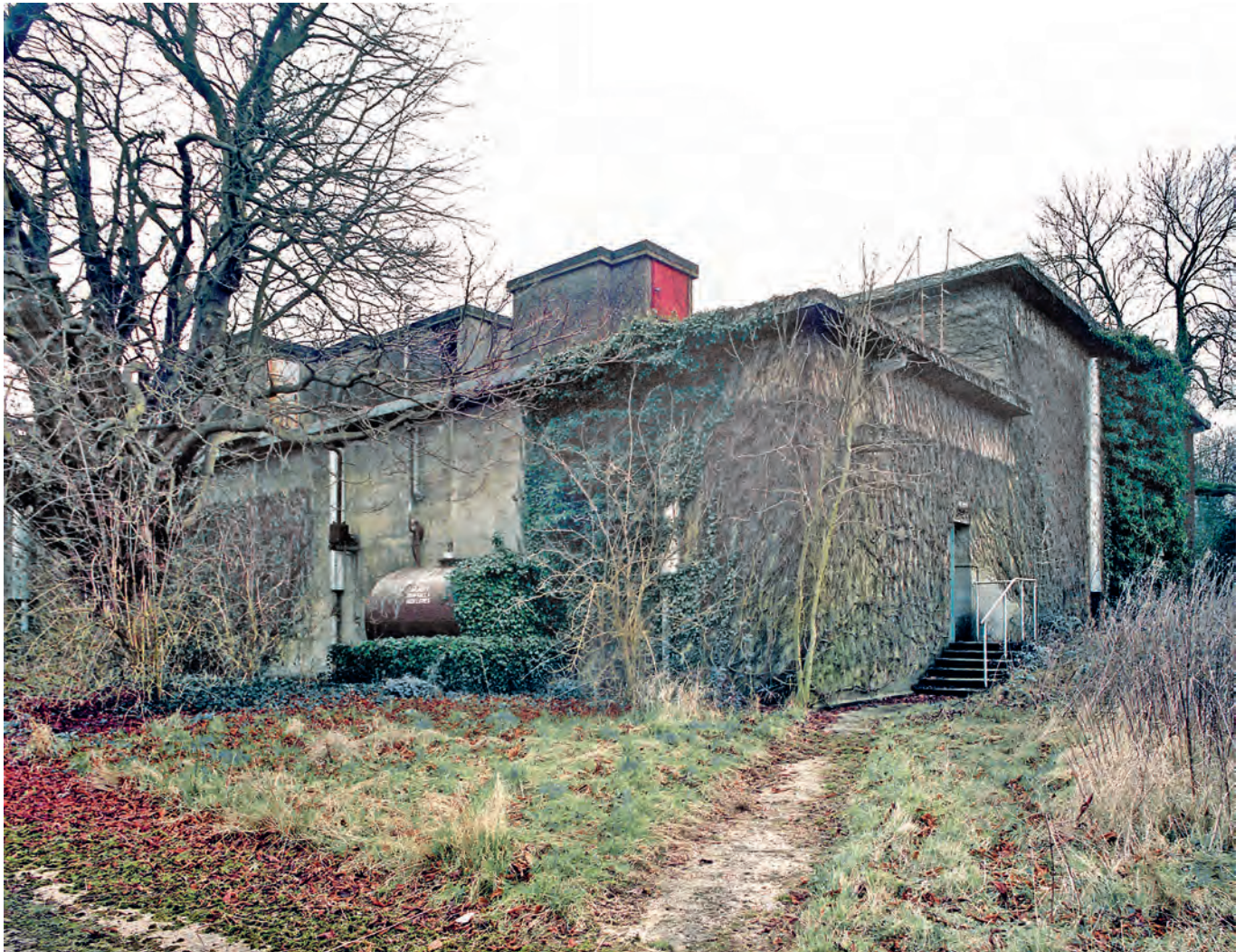
The entrance to the bunker in 2001, before the site was redeveloped. The two-storey extension seen to the rear effectively tripled the size of the bunker; increasing its staff capacity from 50 to over 200. Photo Nick Catford
